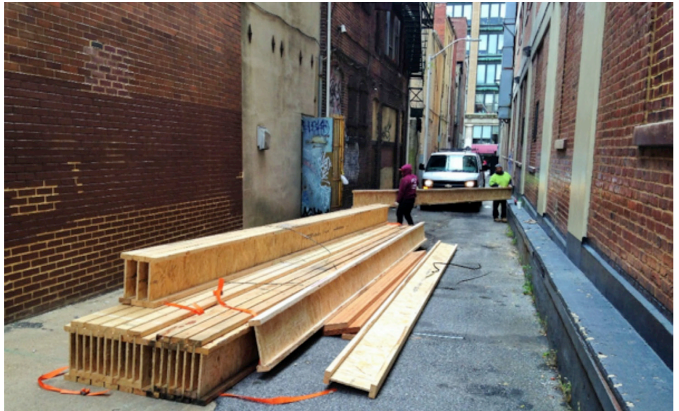
Men carry joists through the alley entrance for a new roof, the first step in renovating the building next to Planned Parenthood in Baltimore for use as a pregnancy center.
