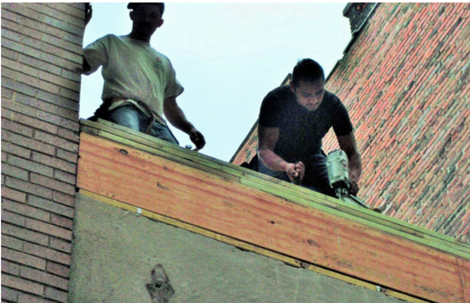
Workers install plywood over roof joists on the alley side of the pregnancy center building.
